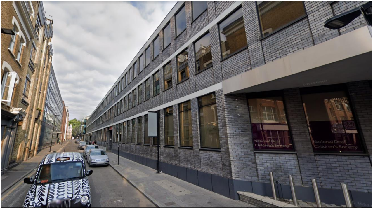
Figure 7: Epworth Street elevation, looking west
