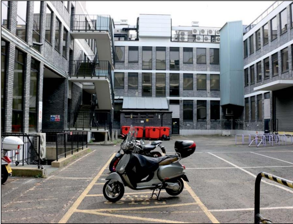
Figure 10: Existing central courtyard
